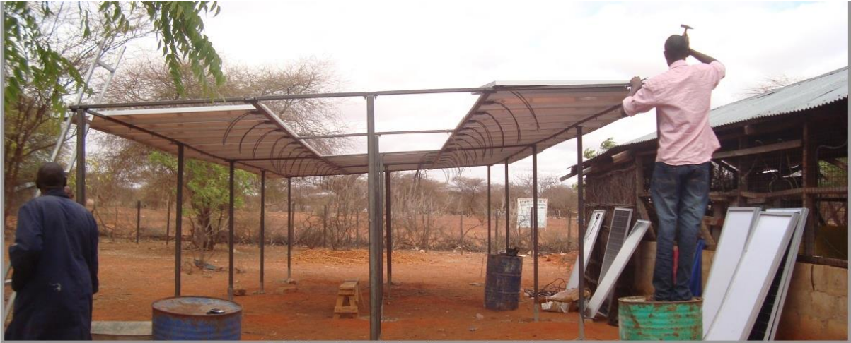
Solar Panels installation ( Damasa borehole
